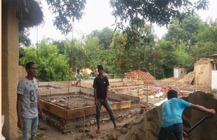
Ongoing Construction at Children Peace home in building Girls Hostel for additional Children. We look forward to accommodate atleast 45 students including Boys and Girls.
